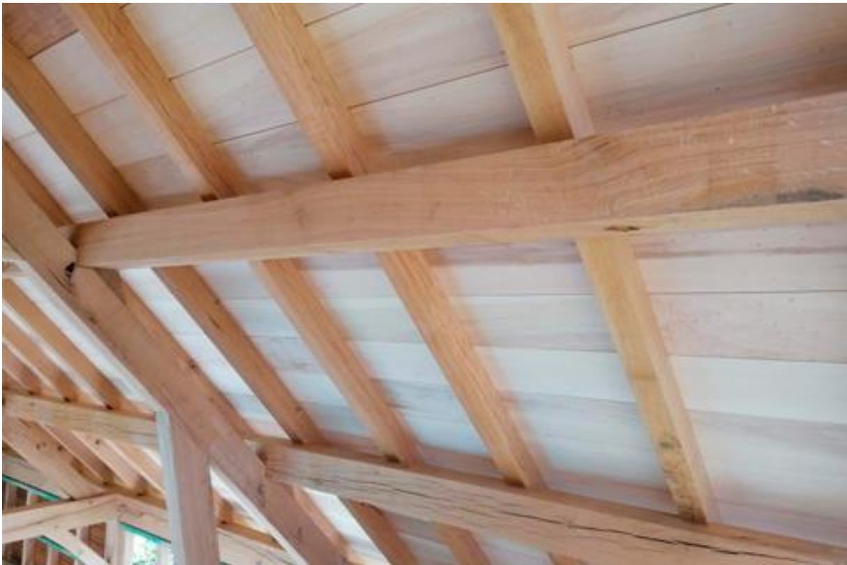
Figuur 20 Dakbeshot (Carpentier, z.d.)
